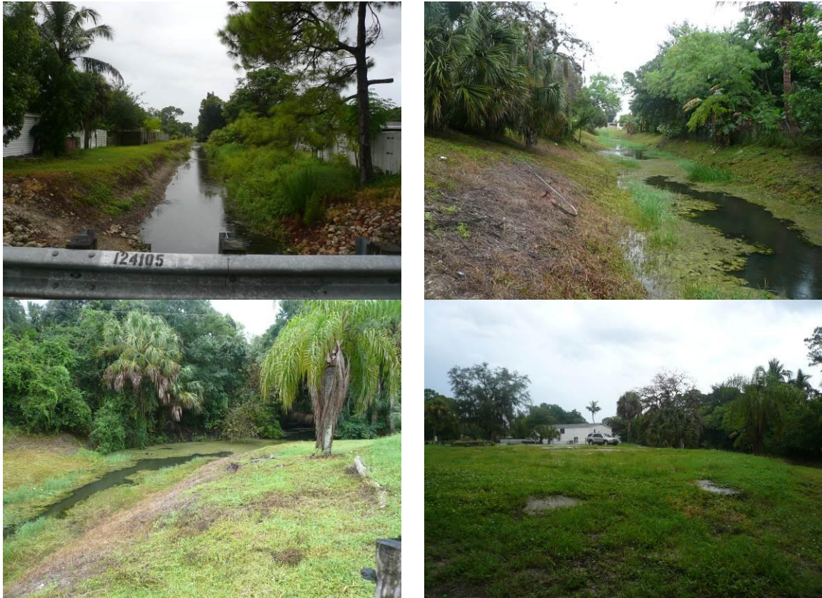
Figure7-24. Potential Site Location, BMP 4
