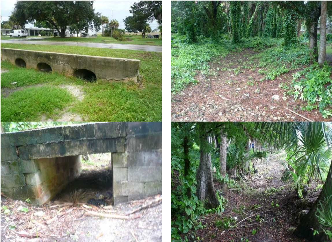
Figure 7-28. Potential Site Location, BMP 6
