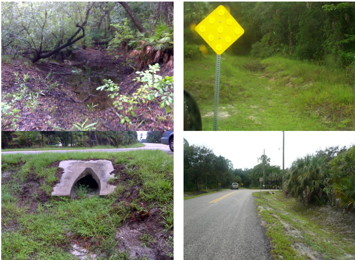
Figure 7-34. Potential Site Location, BMP 9
